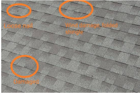
Mechanical damage to shingles.
