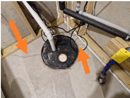
Shrinkage crack. Monitor for any changes in size.
