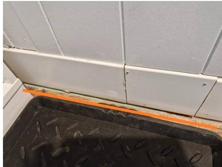
Separation either due to improper installation or the home settling.
