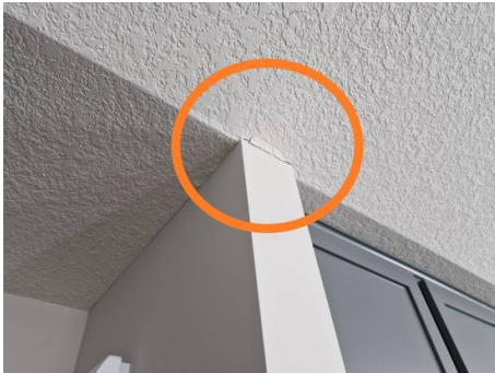
Cracking, possibly due to the property settling. Monitor for a change in color around the edges and crack size.
