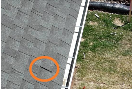
Shingles improperly installed. Possible nail pop pushing shingle up. Also, shingles arched and hanging over the gutter.
