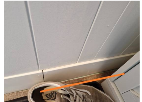
Separation either due to improper installation or the home settling.
